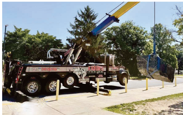
Aaron’s Towing placing the 3.5 ton rock at the school after transport from the quarry.
